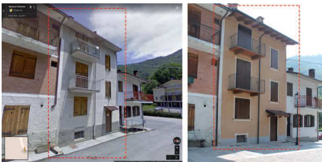
Figure 5 Comparison of the building aspect before and after the recovery intervention with the contributions of measure 322 in the village of Baracco - Roccaforte di Mondovì (CN)
