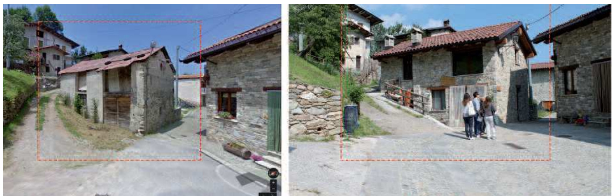
Figure 7 Comparison of the building aspect before and after the recovery intervention with the contributions of measure 322 in the village Baracco (Roccaforte di Mondovì) ( https://www.google.it/maps/@44.2755529,7.749961,3a,90y,334.18h,94.37t/data=!3m6!1e1!3m4!1s5jChC4x2NLXgOYI-AxsvHQ!2e0!7i13312!8i6656 ).
